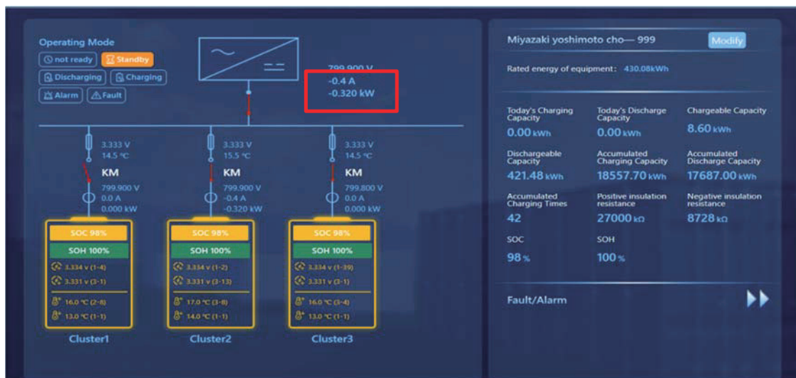
Fig. 14: SCU Monitoring showing charging power limit at 98% SOC
